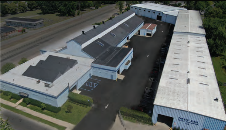
1819 Starr Avenue Warehouse with 25,000 sq. ft. addition.
